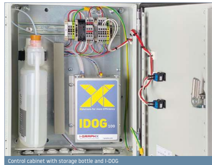
Control cabinet with storage bottle and I-DOG
