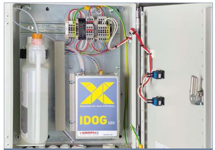
Control cabinet with storage bottle and I-DOG
